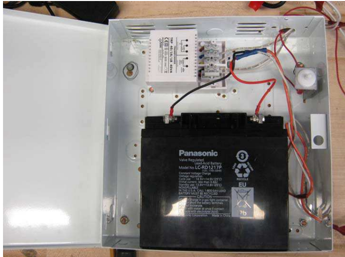
Photo 8: TRP 40/16/18 Transformer and LC-RD1217P Battery with Enclosure
